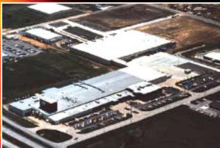
The EnerSys® plant in Warrensburg, Missouri covers 32,000 square feet and is situated on 33 acres.
