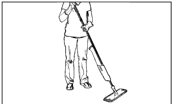
Figure 6. Applying floor finish with Flat Mop (optional)
