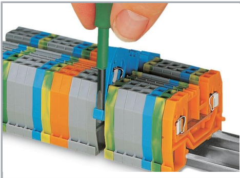
Removing a terminal block from the assembly.
