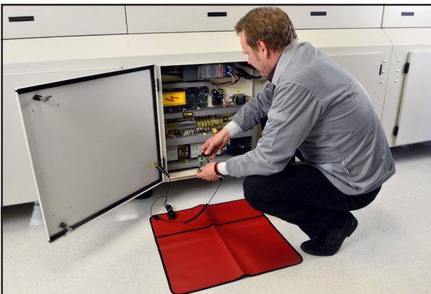
Figure 1. Proper field service ESD control.
