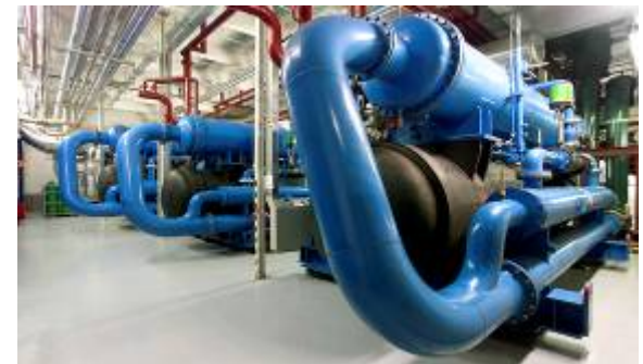
30 MW cooling capacity
