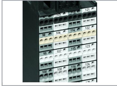
Insulation stop is in place.
