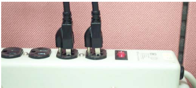
Figure 3.2: Power cord plugs should have same orientation in the socket/ 插座上电源线方向相同 / 插座上的電源線方向應相同
