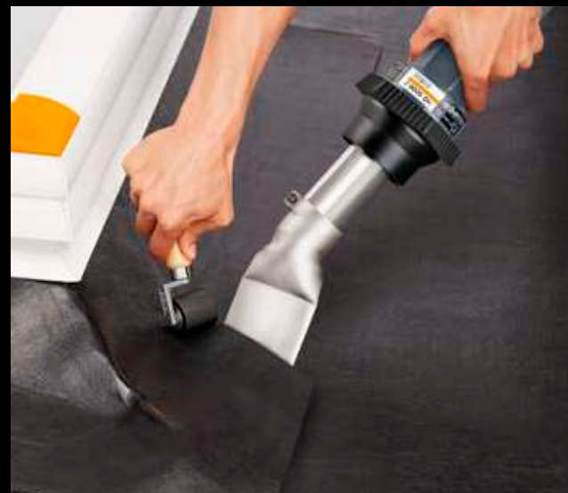
Overlap welding on a light dome.
