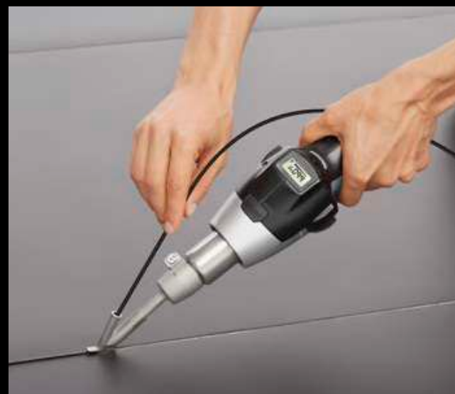
Welding linoleum floors.
